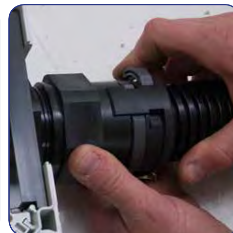
The combined gland and compression fitting is then tightened up to make the internal compression seal on the outer cable sheath
